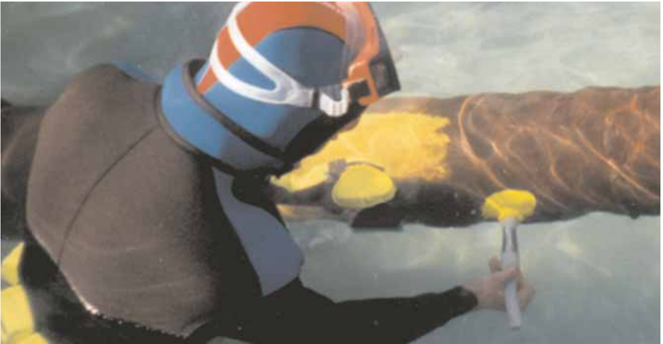
Above: Brush application in the splash zone
