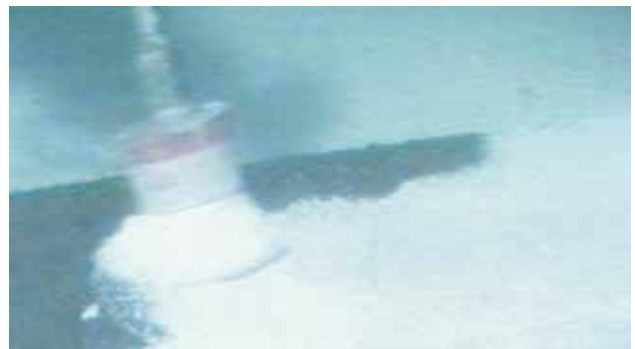
Above: Alocit coatings were applied through running condensation on pipes carrying cooling water under the Petronas Towers in Kuala Lumpur
