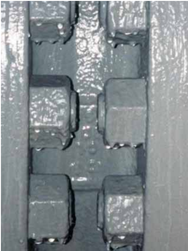
Above: Alocit coatings were applied through running condensation on pipes carrying cooling water under the Petronas Towers in Kuala Lumpur
