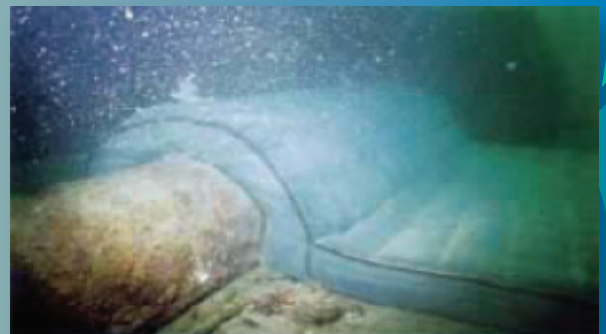
Stabilization mattress on 24" pipeline
