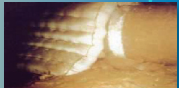
Stabilization mattress on 250mm Thick
